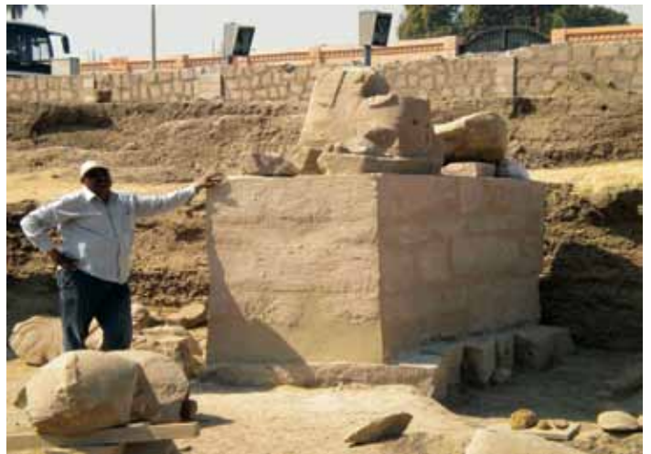
Sphinx being restored on sphinx road
