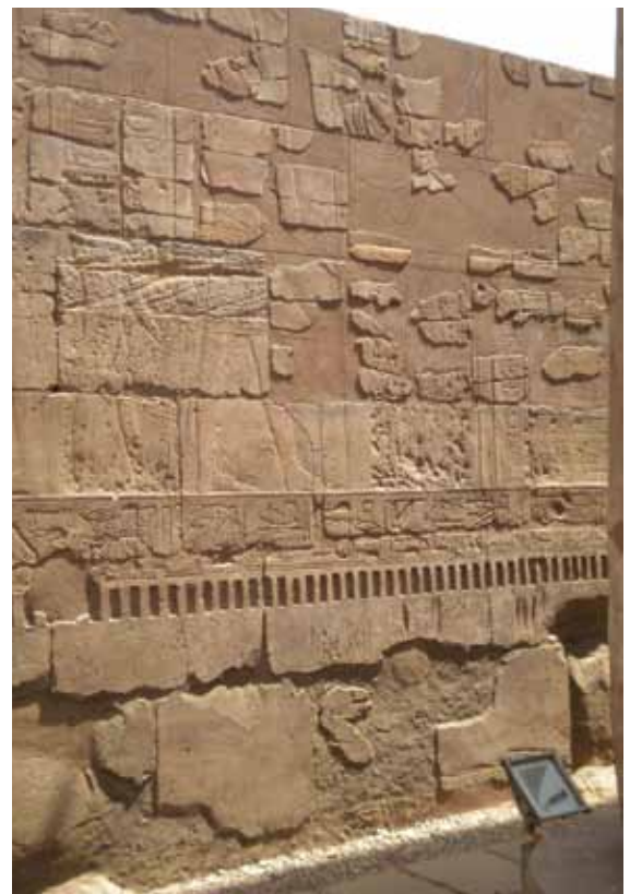
The finished, restored Amenhotep III wall
