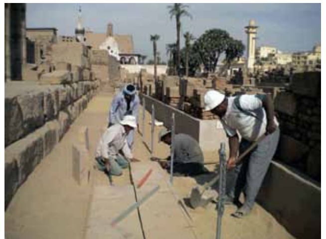
Luxor Temple blockyard open-air museum path construction
