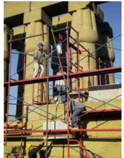
Amenhotep III outer wall slab construction
