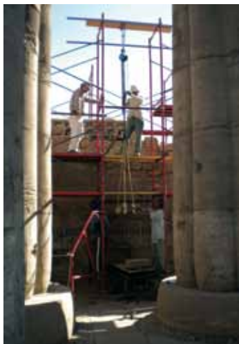
Amenhotep III wall construction
