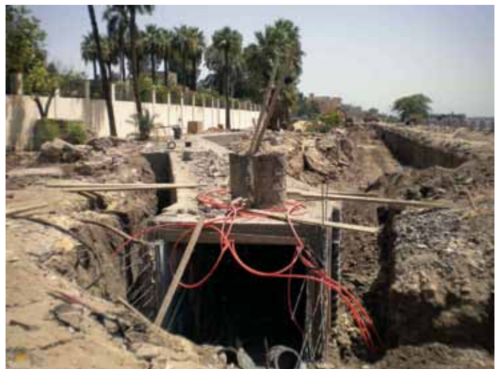
Corniche service tunnel and riverbank construction, June 2010
