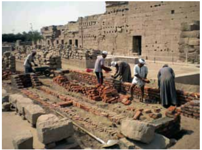
Display mastaba construction
