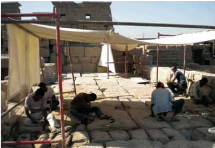
Khonsu Temple roof work
