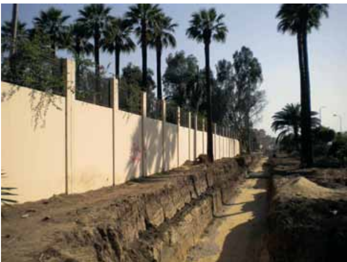
Service tunnel trench outside Chicago House, March 24, 2010
